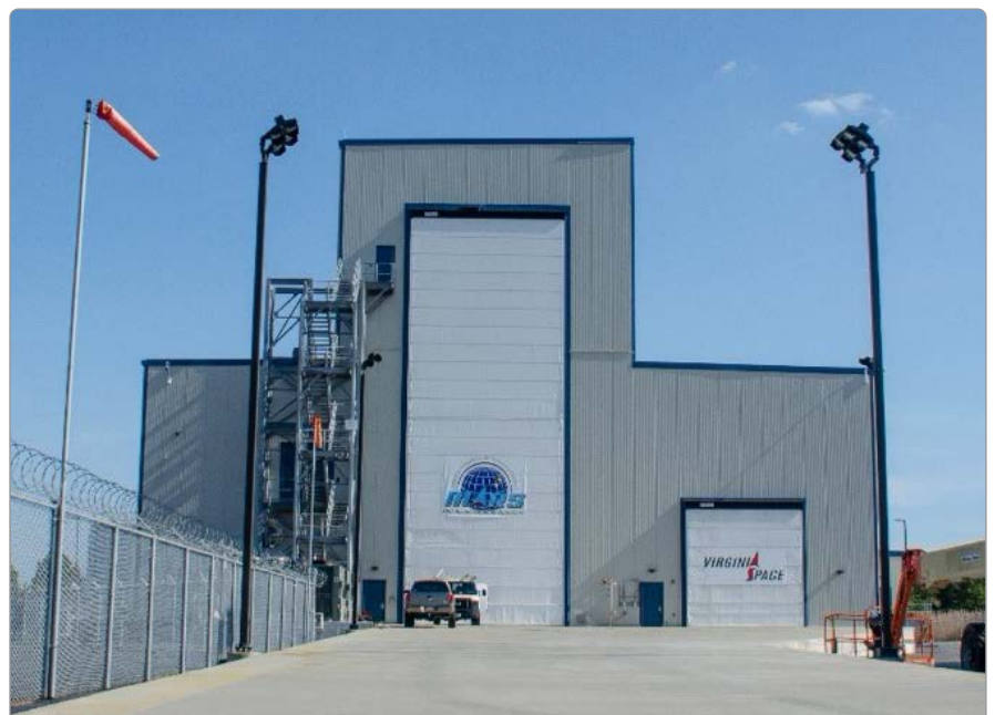
Figure 26 | Mid-Atlantic Regional Spaceport (MARS) Payload Processing Facility (PPF).
