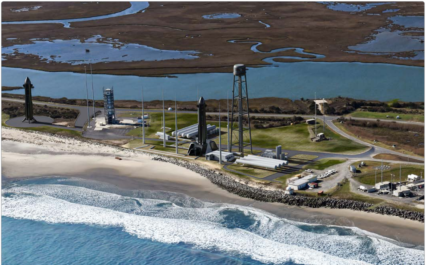
Figure 24 | A Render Of Rocket Lab Launch Complex 3 In Full Operation
