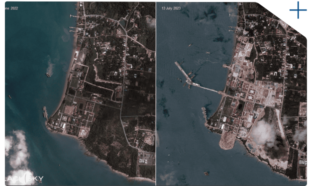
Sihanoukville / Cambodia June 2022 (on left) and July 2023 (on right), images show the newly created deepwater angled pier at Ream.
