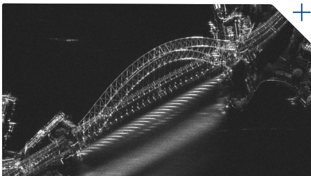
Sydney Harbour Bridge
